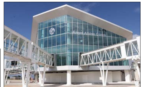
Terminal of the Ángel Albino Corzo International Airport
